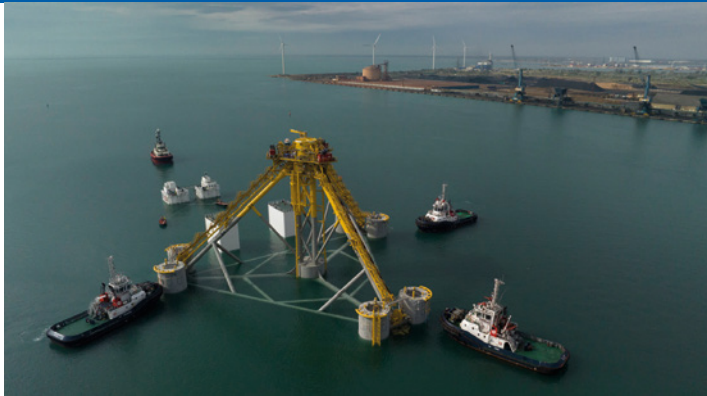
Figure 2. The Provence Grand Large (PGL) floating offshore wind farm (FOW).
